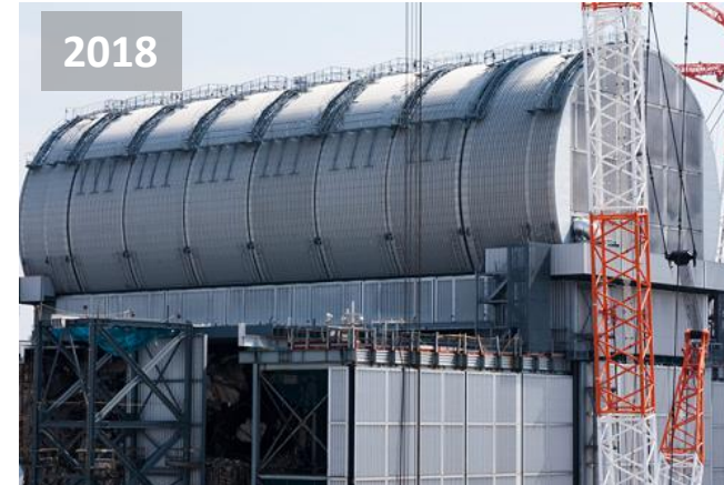
Installation of building cover and remote fuel handling system
