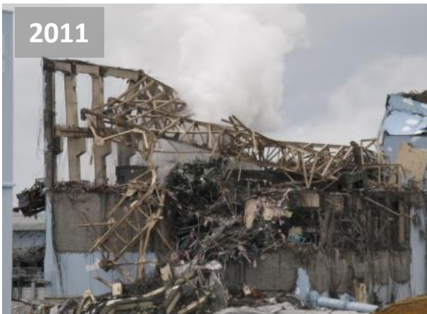
Operating floor damaged by hydrogen explosion (appearance)
