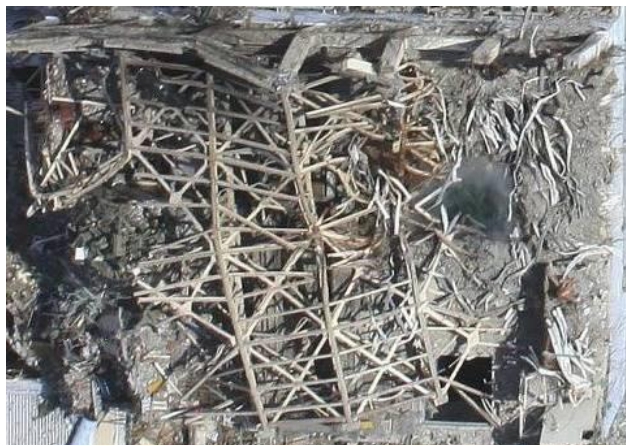
Operating floor damaged by hydrogen explosion (from the above)
