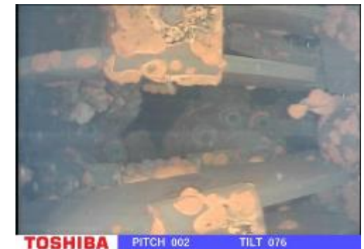
Beneath of CRD housing
